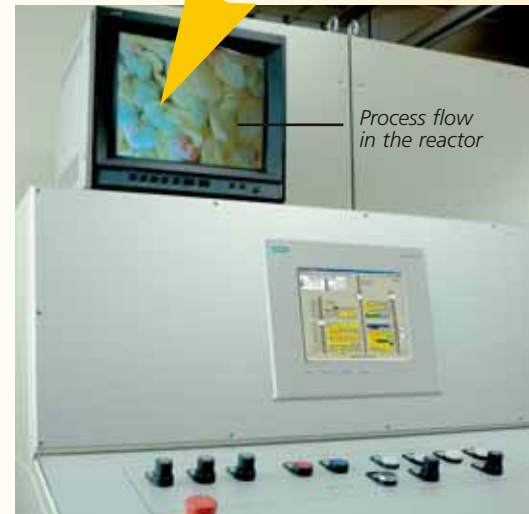
Pictures taken by the camera are shown on a monitor screen in the control room situated outside the Ex hazardous area
